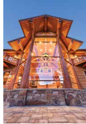
Schafer's Glass Forest window system features 23-foot-tall cedar tree trunks that are flared at the bottom for a design that's as striking from the outside as it is from the interior. Although the cabin is less than 4,000 square feet, the expansive glass in the great room makes it feel much bigger.
